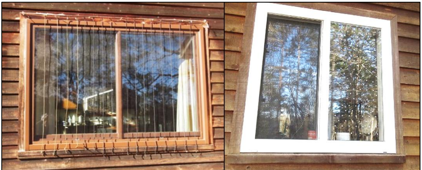
Examples of bird-friendly window options from Pam Stewart, bungee cord method (left) and Feather Friendly sticky dots (right)
